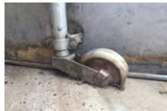
Conventional heavy-duty wheels wear down quickly due to continuous use and the enormous forces of up to 200 kg per wheel acting on them. The blocked wheels scrape across the bottom as the rake rotates. This damages the bottom of the secondary clarifier, which only becomes visible when the tank is
