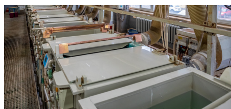
Etching, plating tanks
